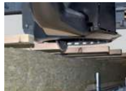
Formatting the roof battens
