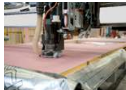
Processing gypsum plasterboard
