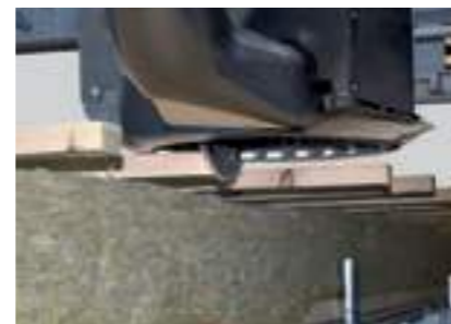
Formatting the roof battens
