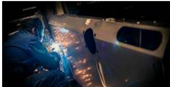
Welding of frame
