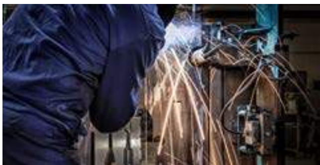
Welding of frame
