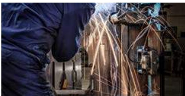
Welding of frame
